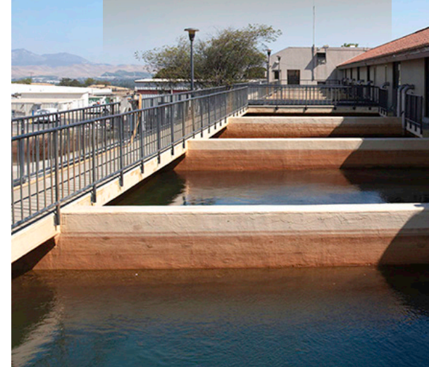
Filters at Del Valle Water Treatment Plant
