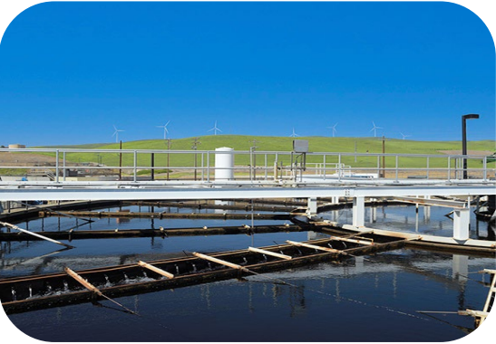
DVWTP and PPWTP HVAC and Improvements
