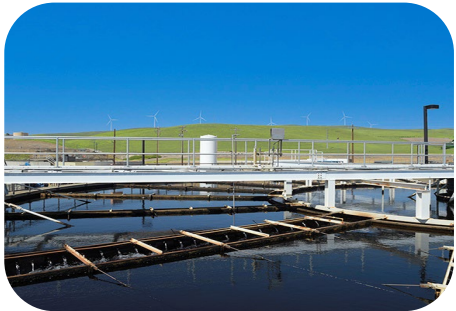
DVWTP and PPWTP HVAC and Improvements
