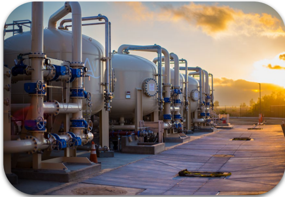
Completion of COL PFAS Treatment Plant
