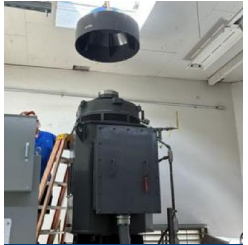
Stoneridge Well Emergency Repair
