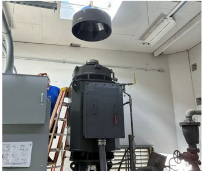
Stoneridge Well Emergency Repair Motor Alignment
