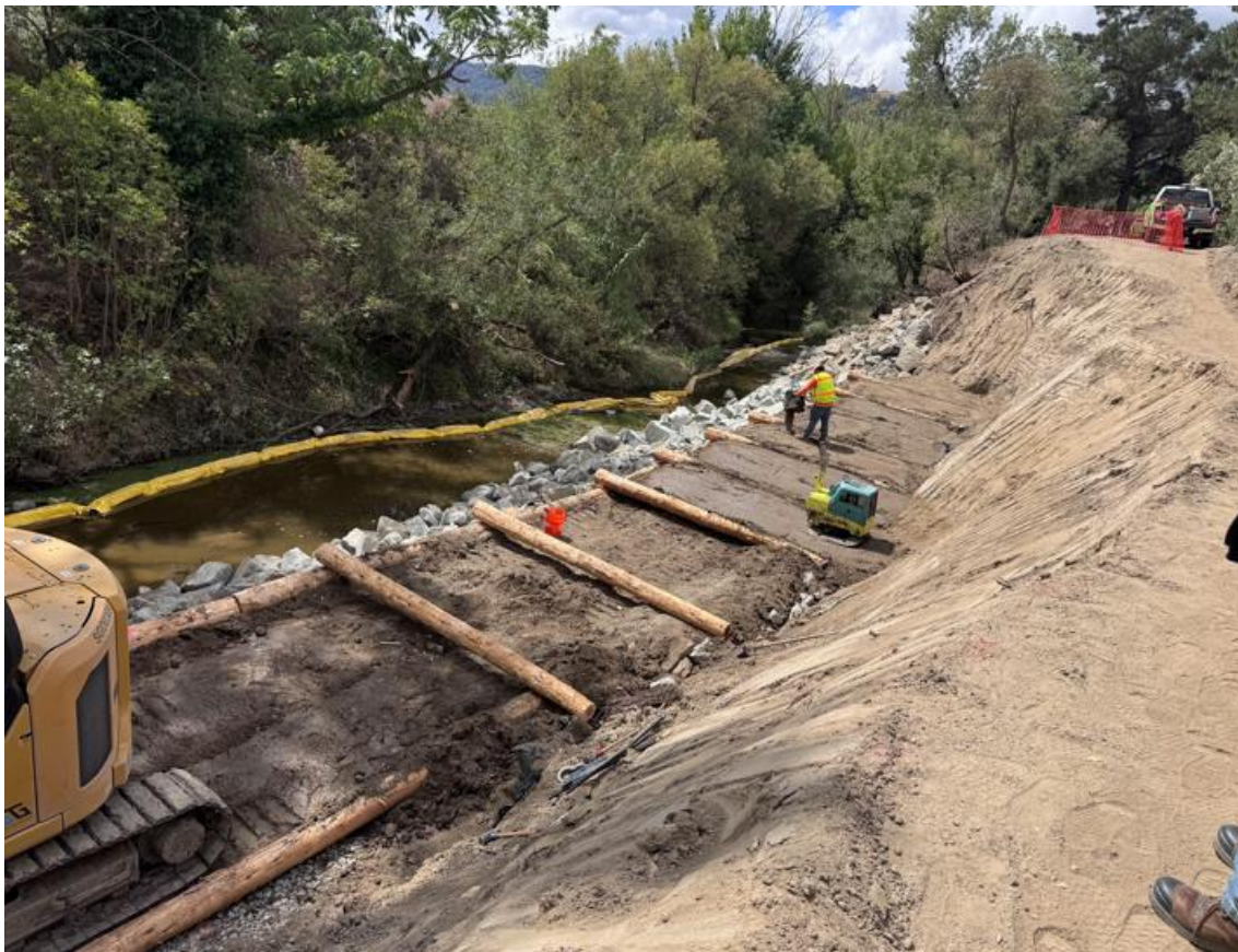
Timber log crib wall under construction at Arroyo del Valle in Pleasanton.
