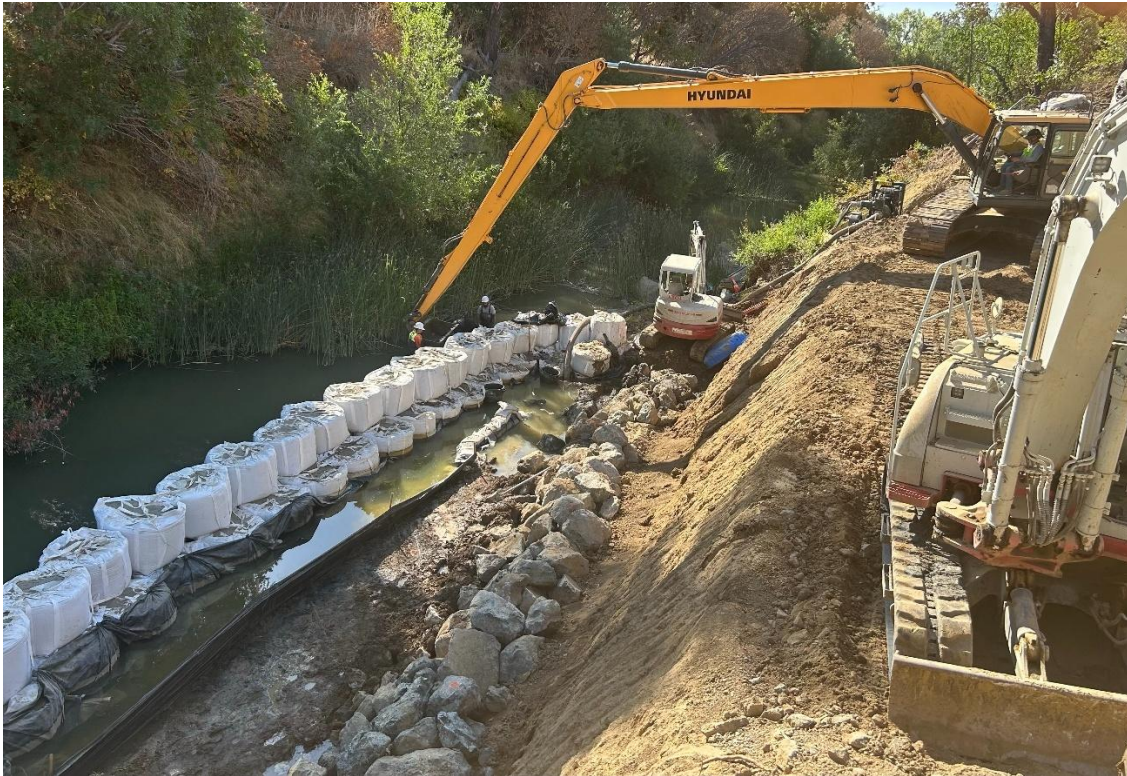
Construction crews install rock slope protection and temporary water diversion measures as part of bank stabilization improvements to restore channel integrity and reduce future erosion at Arroyo de la Laguna near Golden Eagle Estates in Pleasanton.
