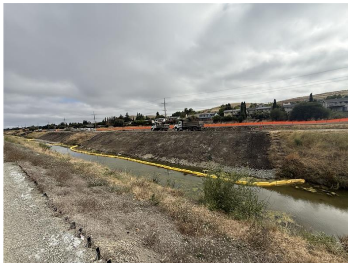
Phase 1 Storm Repair Project construction activities.
