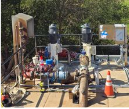
DVWTP Booster Pump Station VFD and Underdrain Pump Station Project - Completion March 2026
