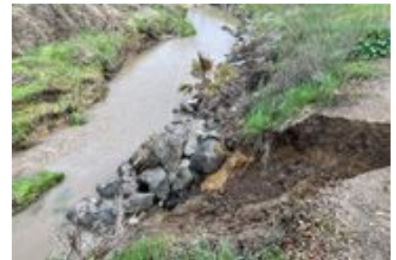
Future Storm Damage Repairs - Line H-N at Vasco
