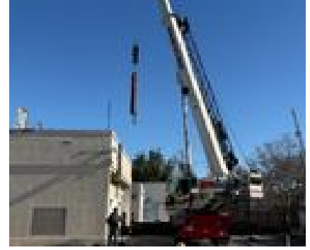
Stoneridge Well Emergency Repair - Well Pump Reinstallation
