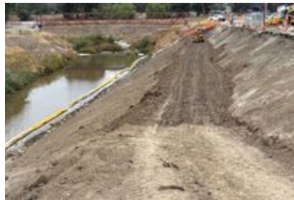
US Army Corps of Engineers Rehabilitation Project
