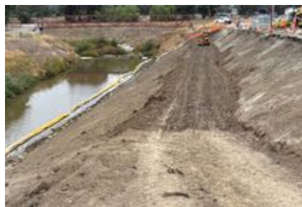
US Army Corps of Engineers Rehabilitation Project
