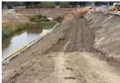
US Army Corps of Engineers Rehabilitation Project
