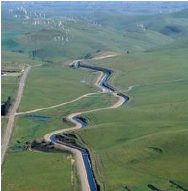
South Bay Aqueduct
