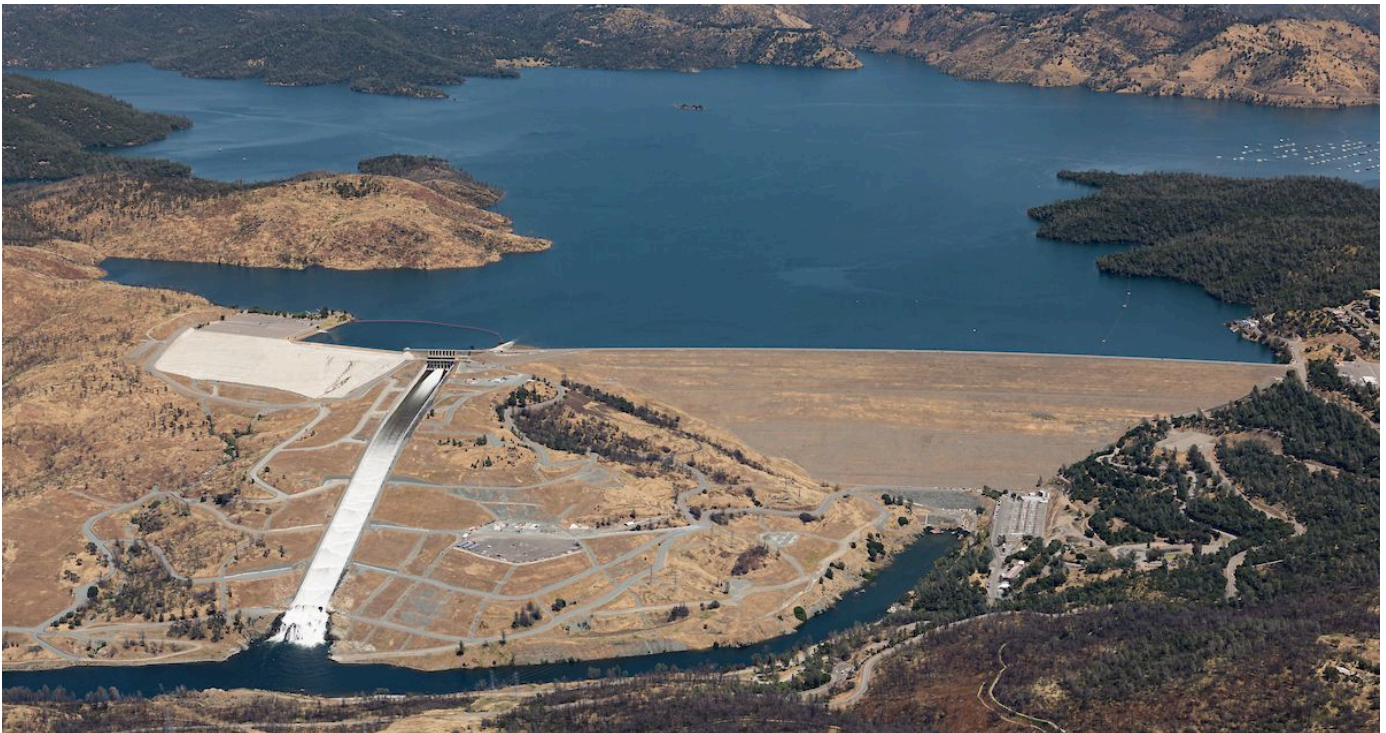
Lake Oroville spillway - May 2025
