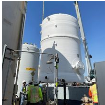
Patterson Pass Coagulant Tank Replacement Project
