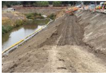
US Army Corps of Engineers Rehabilitation Project
