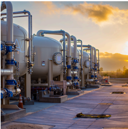
Chain of Lakes PFAS Treatment Facility - Completion September 2026
