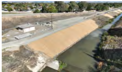
US Army Corps of Engineers Rehabilitation Project Line G – Arroyo Mocho in Pleasanton
