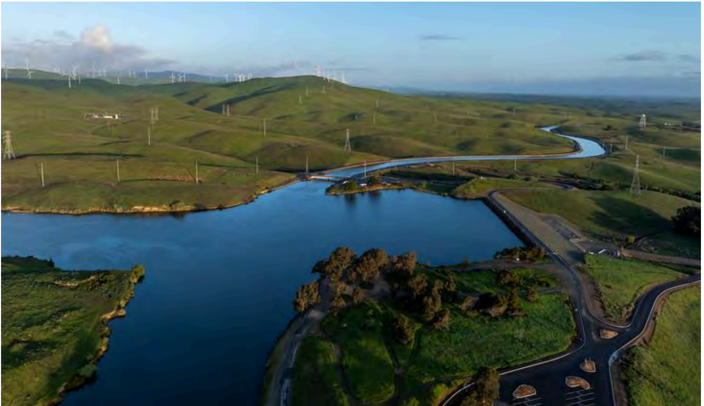
Bethany Reservoir, Alameda County - March 2026
