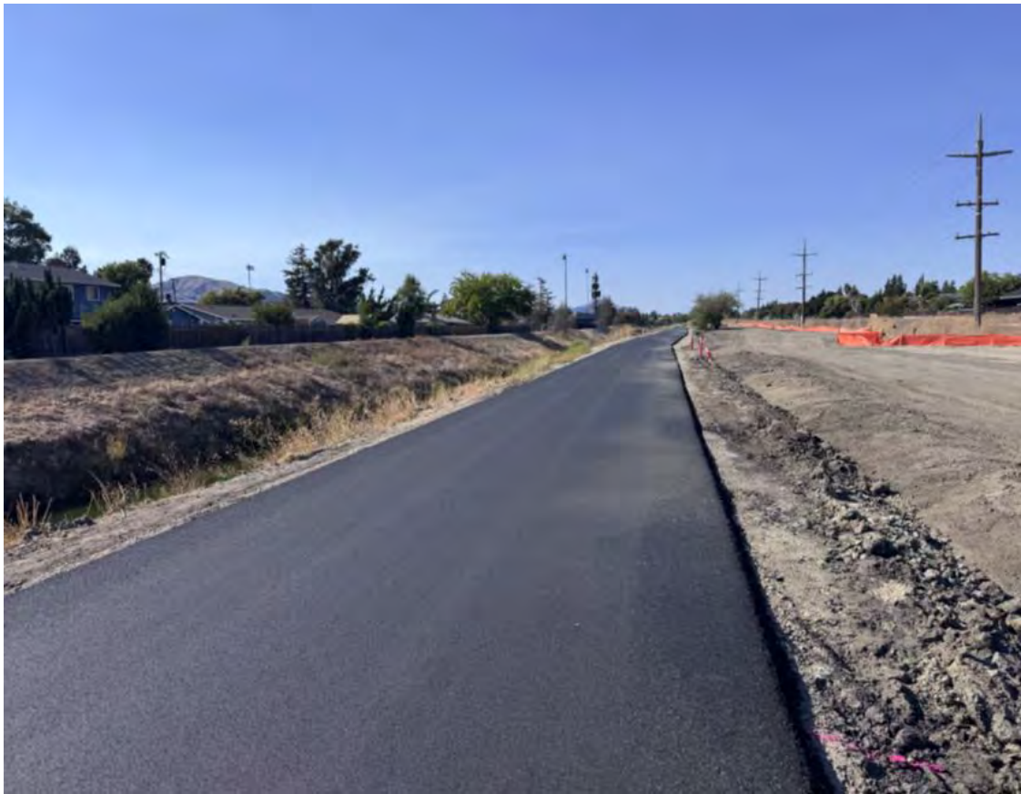
Restored segment of the Iron Horse trail along South San Ramon Creek in Dublin, now open to the public
