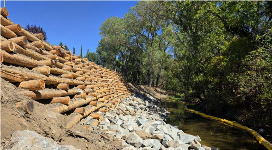
Completed timber-log crib wall at Arroyo del Valle in Pleasanton
