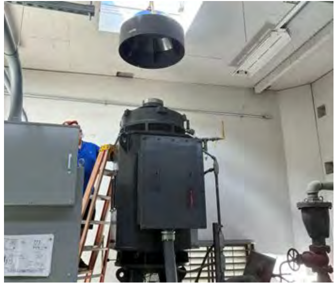
Stoneridge Well Emergency Repair Motor Alignment
